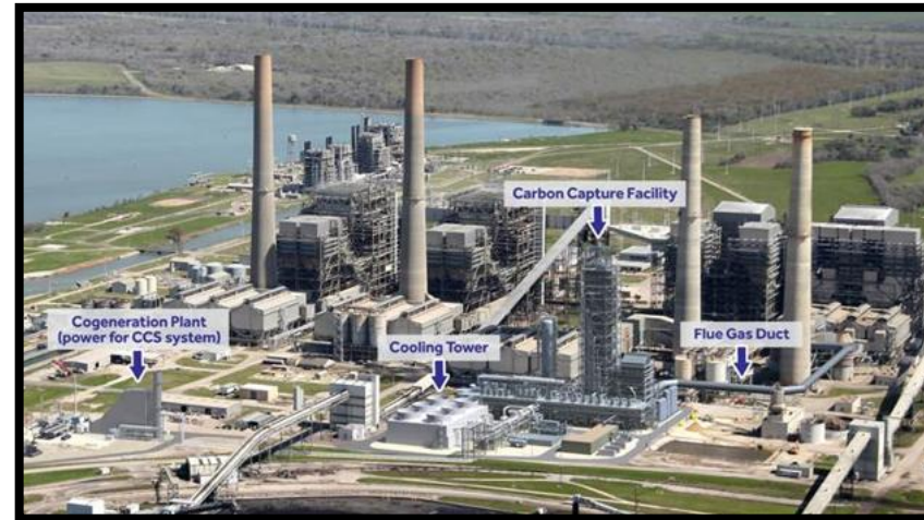
Petro Nova Carbon Capture Plant
