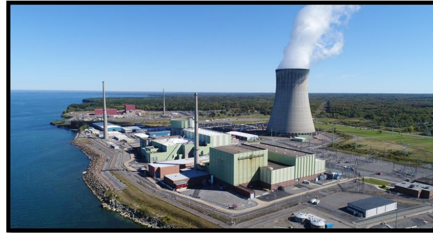
Nine Mile Point Nuclear Station / Hydrogen
